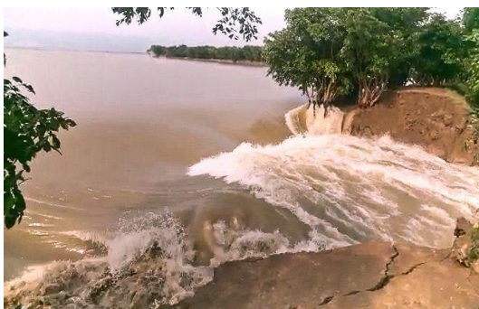
Image 6 Water enters in to Tanguar Haor dam in Tahirpur Upazila (adapted from Desk Report, 2022).
