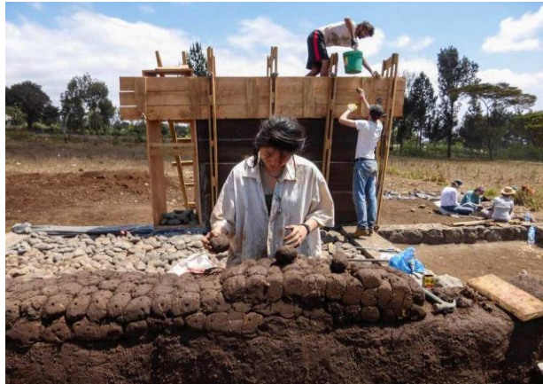
Figure 8: Typical Cob wall under construction
