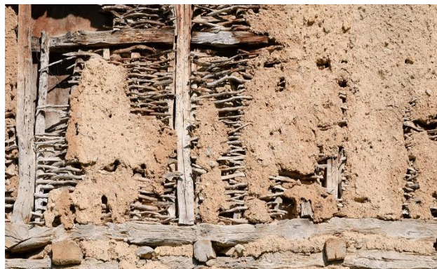
Figure 9: Typical Wattle and Daub Wall
