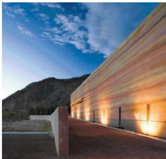
Figure 14: Typical image of layered REW found at Osoyoos Indian Reserve in British Columbia, Canada (Gramlich, 2013)
