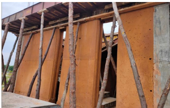
Figure 10: Typical Poured Earth Wall
