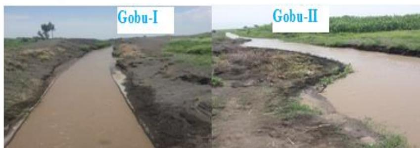
Figure 4.2 Gobu-I and Gobu-II main canal sedimentation and canal leakage
