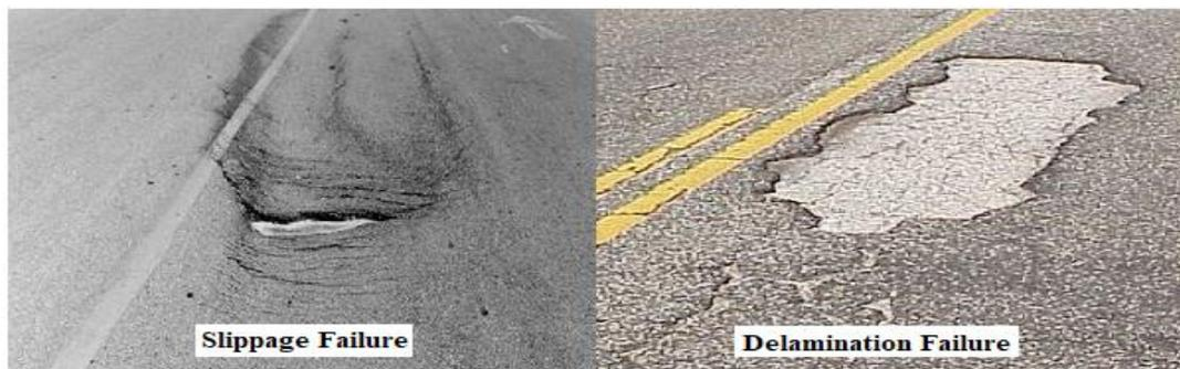
**Figure 1** Premature Failure Due to Bond Interface, (Kulkarni, 2004)
