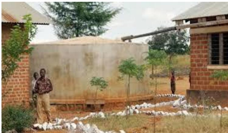
**Figure 3** Rain water harvesting from roof tops
